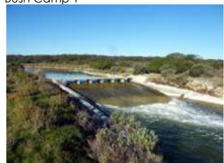
Head north along the Nukan Kungun Hike to the weir. This is the point at which water from the South-east Draining scheme enters the Coorong
